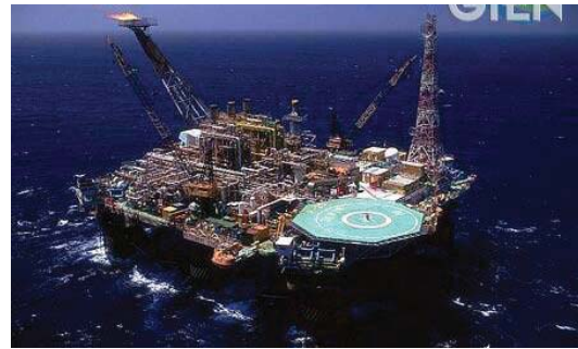
Figure 1 – Typical SS production unit
