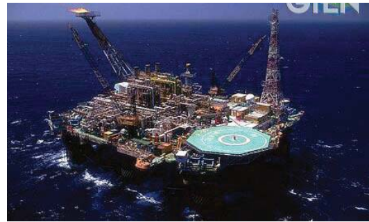
Figure 1 – Typical SS production unit
