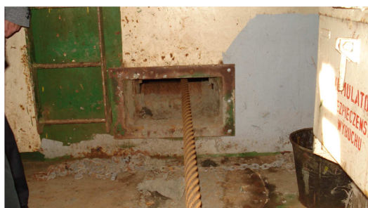
Figure 3: Anchor rope going through the bulkhead from the locker to the hold
