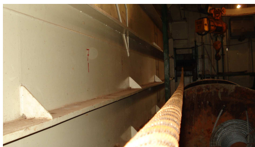
Figure 4: Anchor rope in the hold seen in the direction from hoisting winch to the locker
