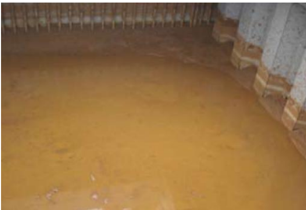
Figure 4: Example of liquefaction
