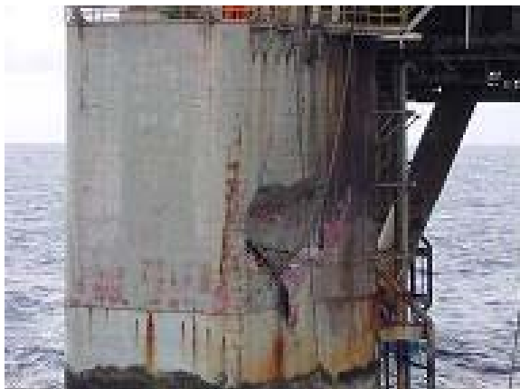
Figure 2 – Semi submersible unit's column hit by a tugboat.
